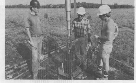
(9112), Dave Lee (9243), Tom Cabe (2312), Lew Bartel, and Ron Jacobson (both 6242) have evaluated CSAMT's effectiveness in locating and mapping the progress of a steam front in a Utah tar sand (host for crude oil that has a tar-like consistency) steamflood operation.
